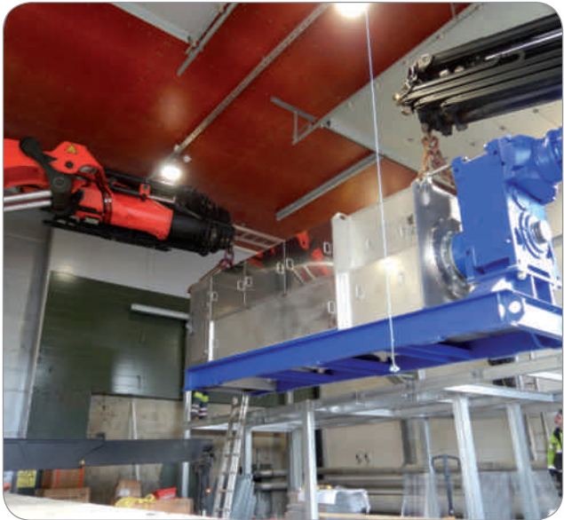
Installation of the screw press – millimeter work.
