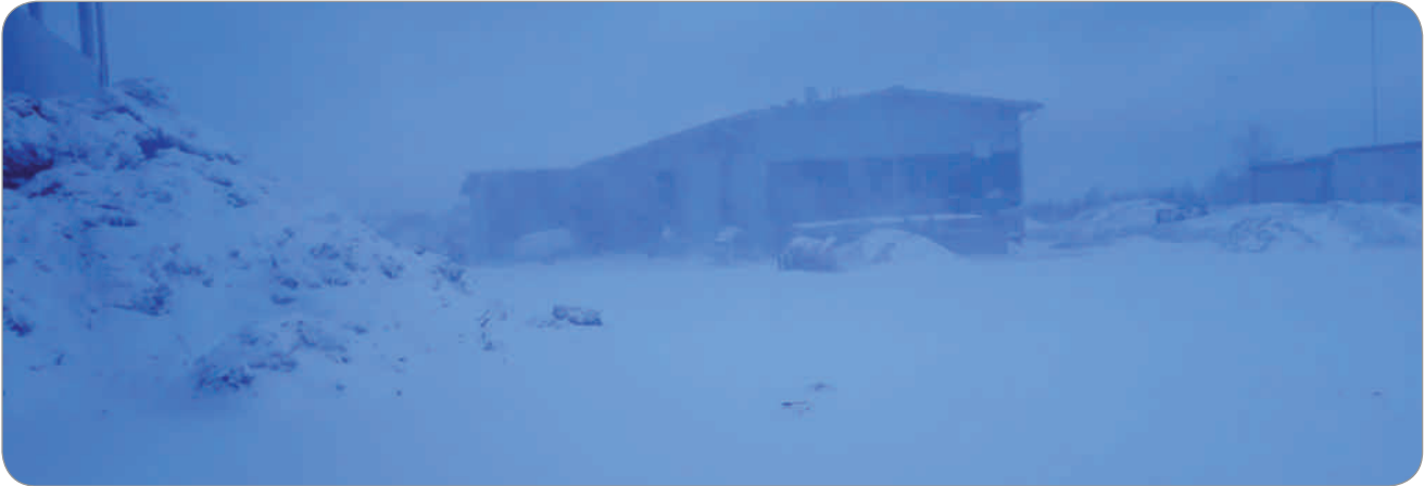
Start of installation despite adverse conditions.
