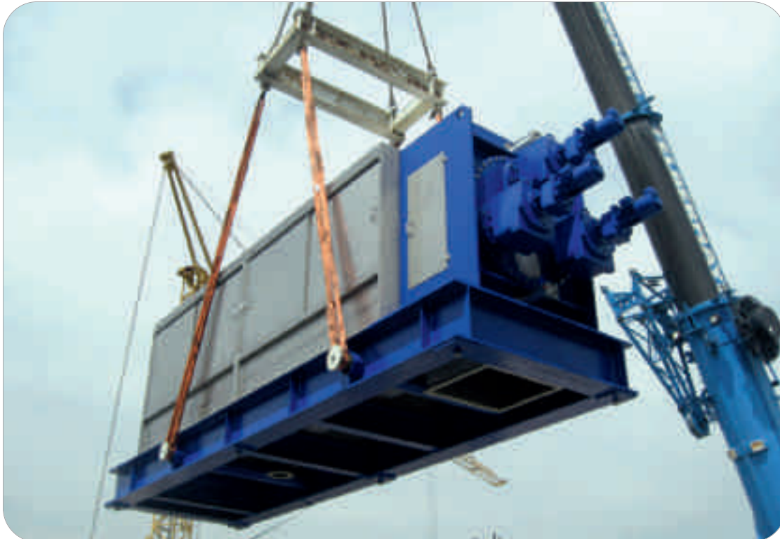
Procedure of bringing the screw press into the new press building
