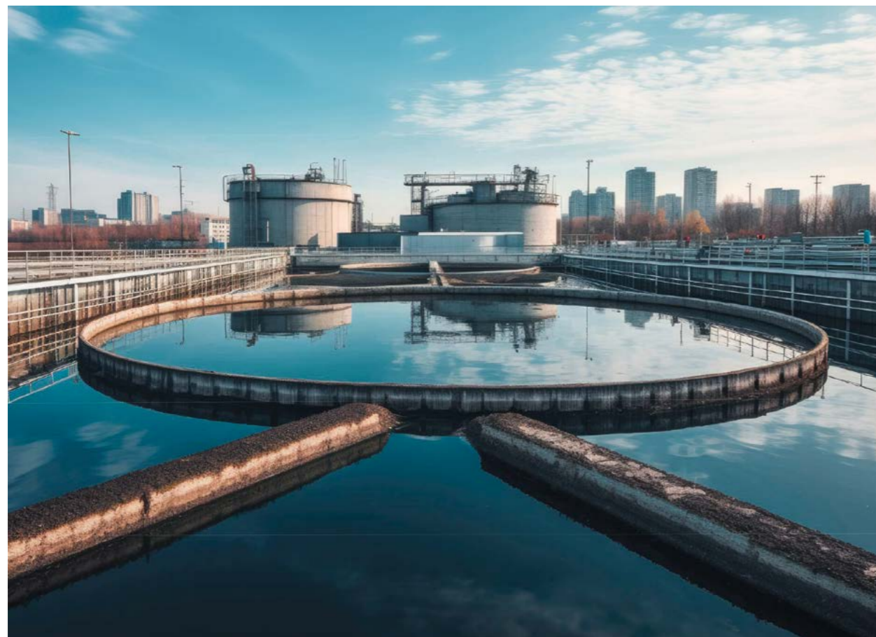
Wastewater treatment plants must be both environmentally friendly and economical to operate.
