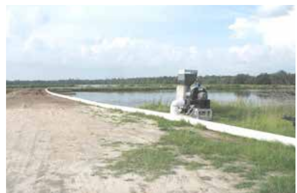
Ecosorb® vapour distribution at a refinery settlement
